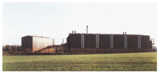
Fig. 1 The new refinery has been built to the north of the existing facilities. The Solvex Building, shown here, houses both process facilities and support units. The process plant is divided into sections, one houses the solvent extraction equipment, another the feed preparation and interstage treatment plant; the metal refining stages are also carried out here
