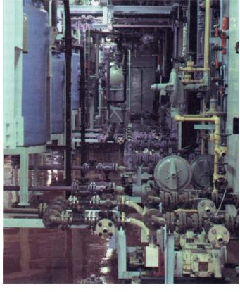
Fig. 4 One hundred and eighty pumps are used to transfer the liquors through the various stages of the extraction process. The use of closed containers minimises the contact of personnel with process materials work commenced immediately and the first noble metal concentrate was fed into the plant in August 1983, since when commissioning trials have continued satisfactorily and are nearing completion.
