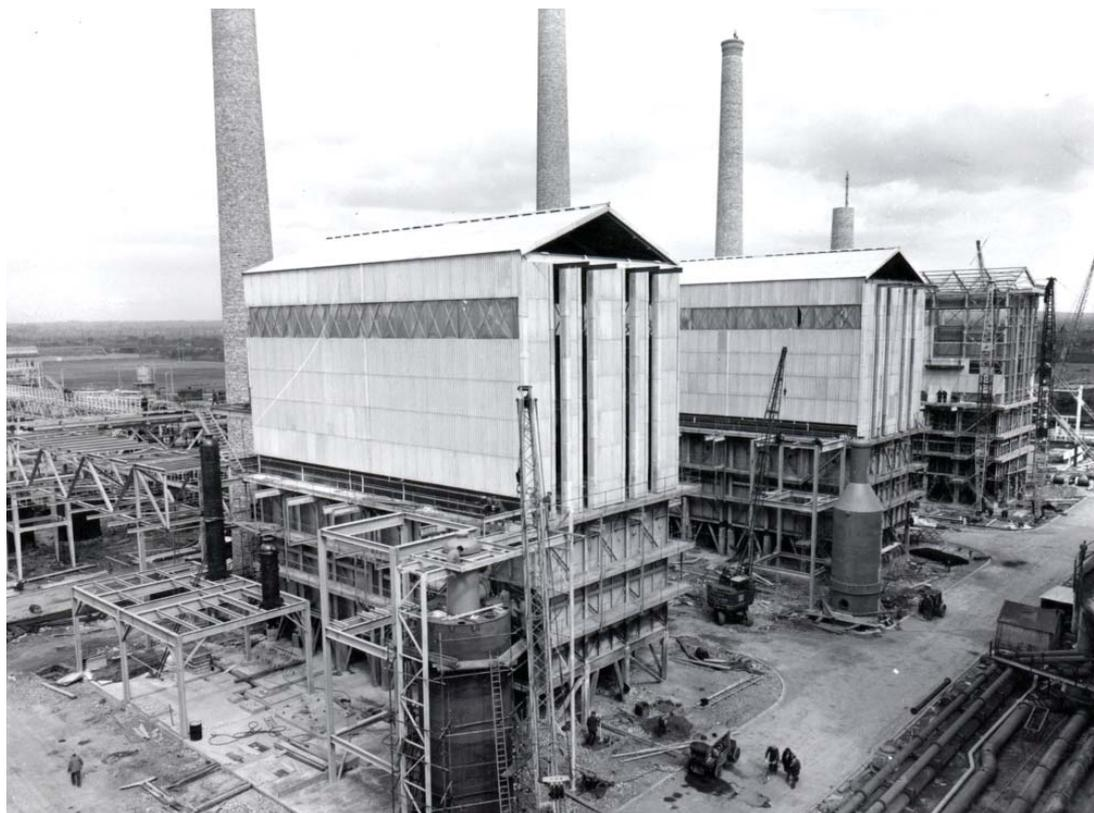
Fig. 3. Construction during early 1962 of the original naphtha steam reformers at Billingham that provided synthesis gas for the ICI Low Pressure Methanol Process. Both the naphtha steam reforming and methanol processes were commercially very successful with several hundred plants being licensed around the world
