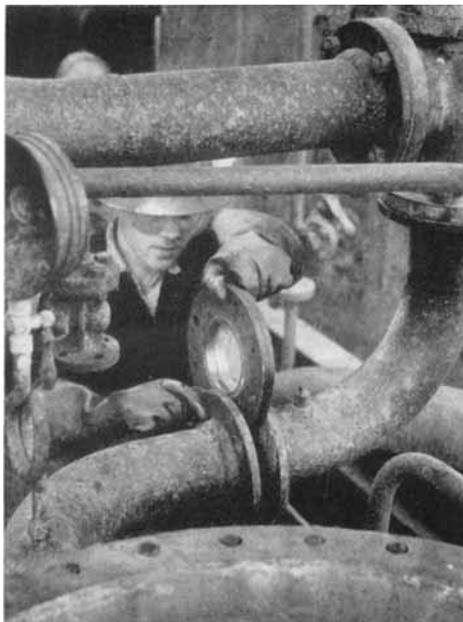
*Fitting a bursting disc assembly into a pipe line*
