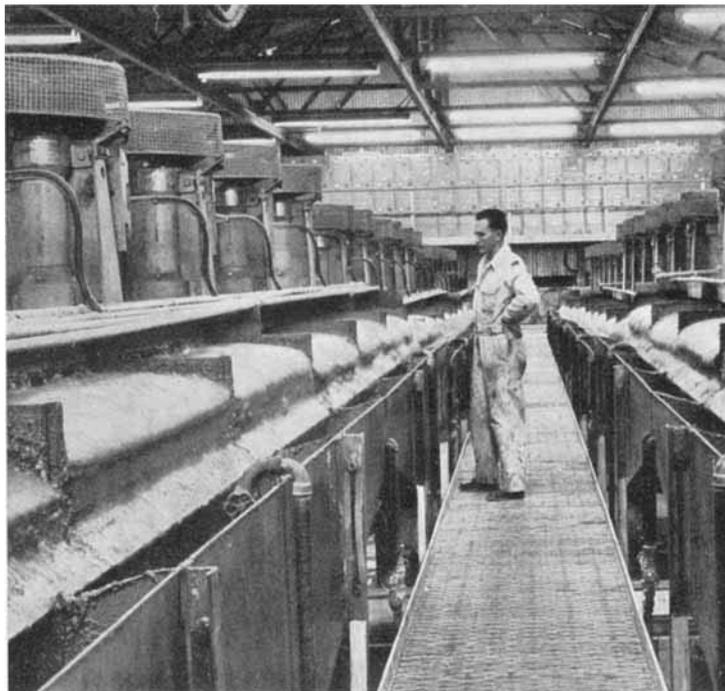
*Banks of cells in the flotation plant. The platinumiferous concentrates are floated off in the white froth shown flowing over the lips of the cells*
