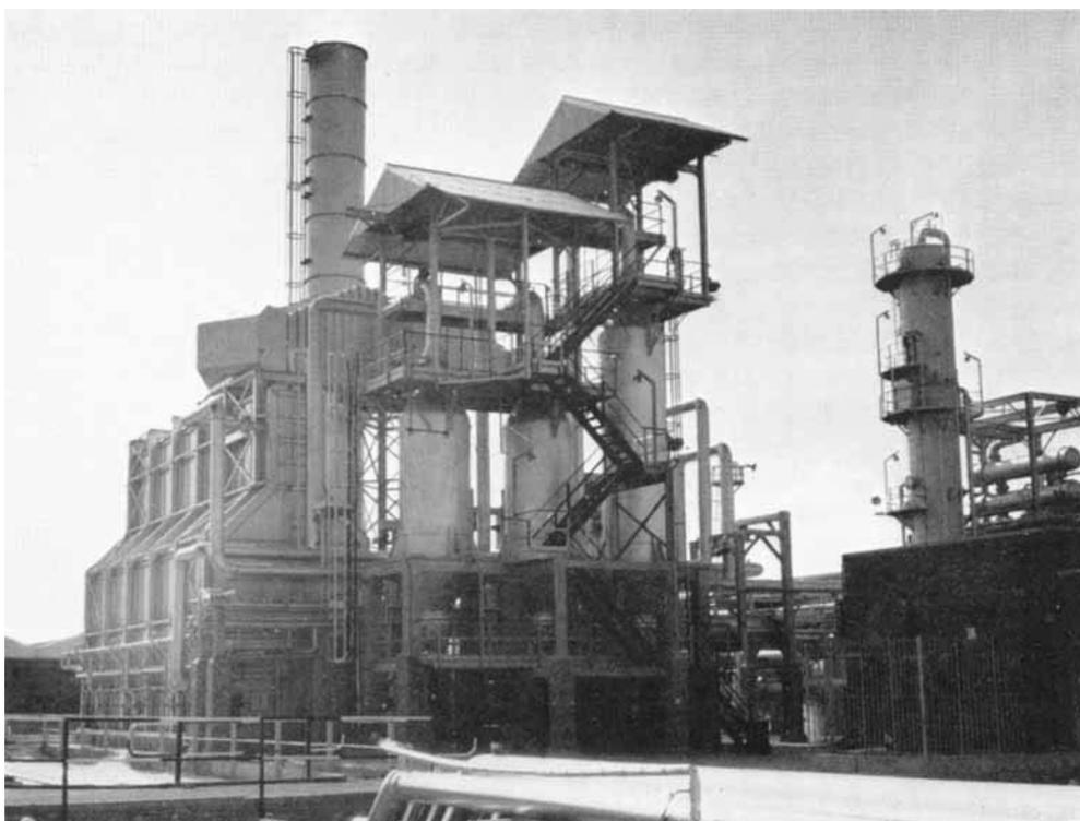
*The reactors of the British Petroleum Company's platformer at the Kent refinery*
