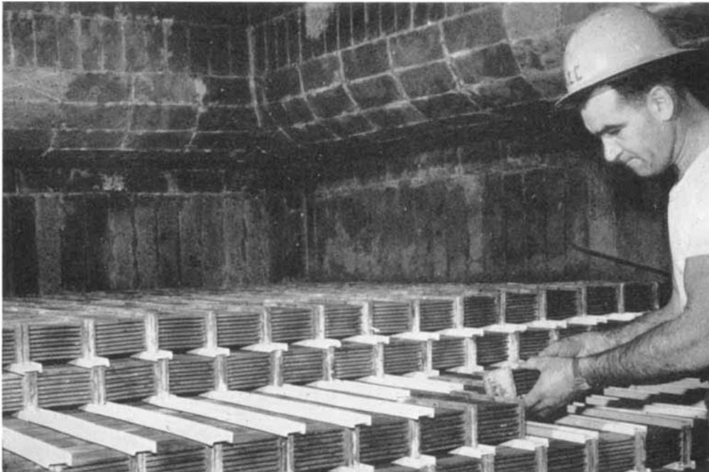
*Fig. 2 Units can be stacked horizontally and vertically to form catalytic beds of any size to meet the requirements of a plant design*
